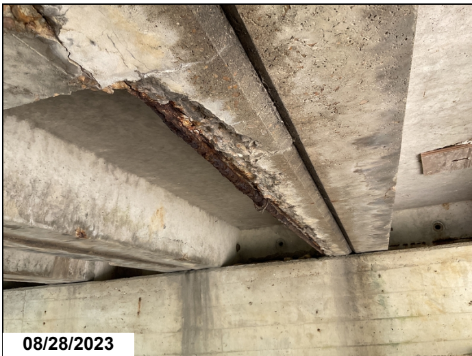
Spalls with rebar exposed with heavy s/l to Girder 7 @ Span 6. 14' of rebar is not adhered to concrete.
