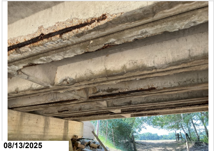
Concrete Precast Units Spalls w/corroded rebar exposed to units @ all Spans. Span 6.
