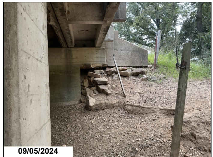
Erosion to wing and right side of abutment 2.
