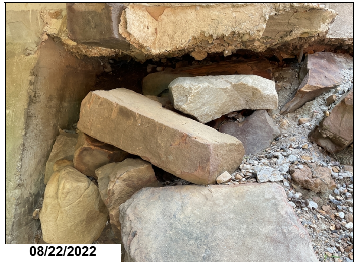
Erosion to Lt & Rt wing @ abutment 2 with Lt wing starting to crack.
