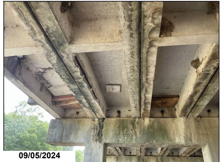
Exposed rebar left leg unit 2 span 4.
