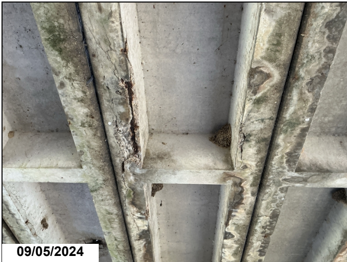
Exposed rebar left leg unit 5 span 4.
