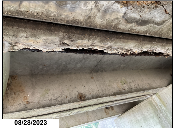
Spalls with rebar exposed with heavy s/l to Girder 2 @ Span 6. 4' of rebar is not adhered to concrete.
