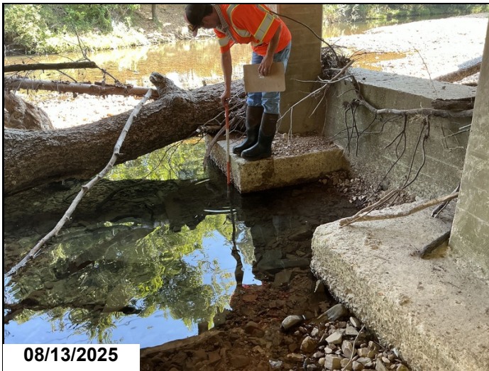
Drift @ Spans 1 - 5. Beginning to cause local scour at bent 4.
