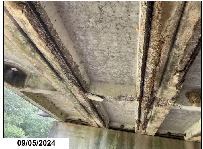
Spalls with rebar exposed with 100% s/l to stirrups @ Girder 2 @ Span 2.
