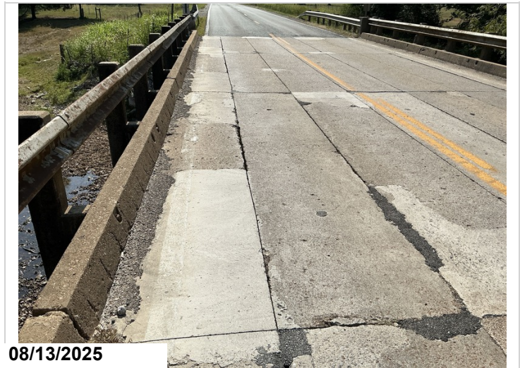
Severe patched concrete areas to units throughout.
