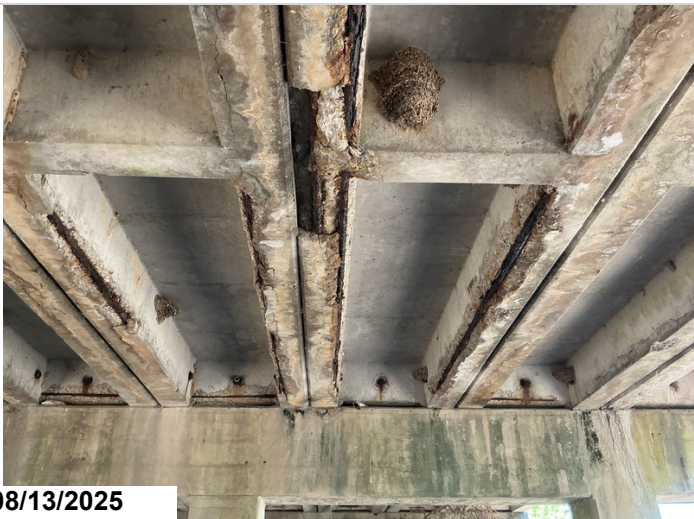
Concrete Precast Units Spalls w/corroded rebar exposed to units @ all Spans. Span 5.
