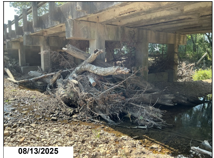
Drift @ Spans 1 - 5. Beginning to cause local scour.
