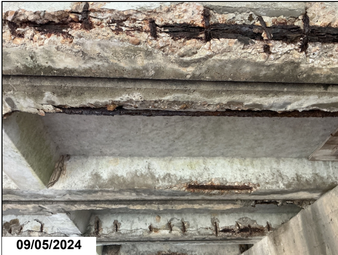
Exposed rebar left leg unit 3 span 1.
