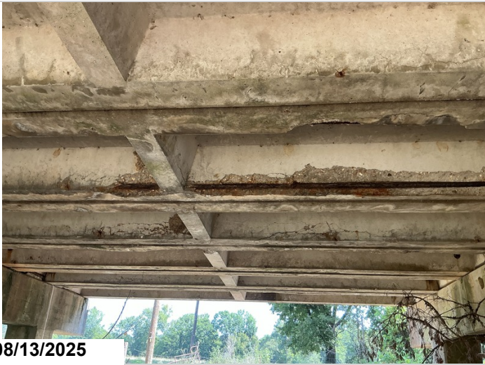
Concrete Precast Units Spalls w/corroded rebar exposed to units @ all Spans. Span 3.
