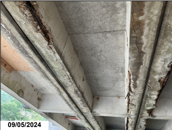
Exposed rebar to left and right leg unit 2 span 6.
