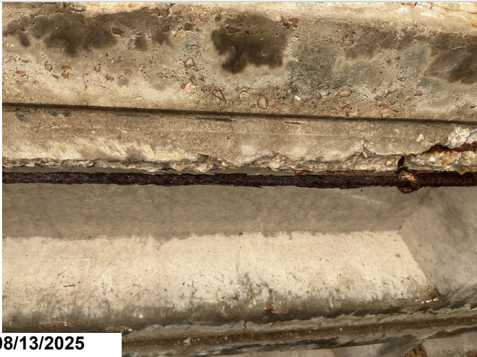
Units that have spalls with rebar exposed that have lost adhesion to concrete: Span 6 unit 6.
