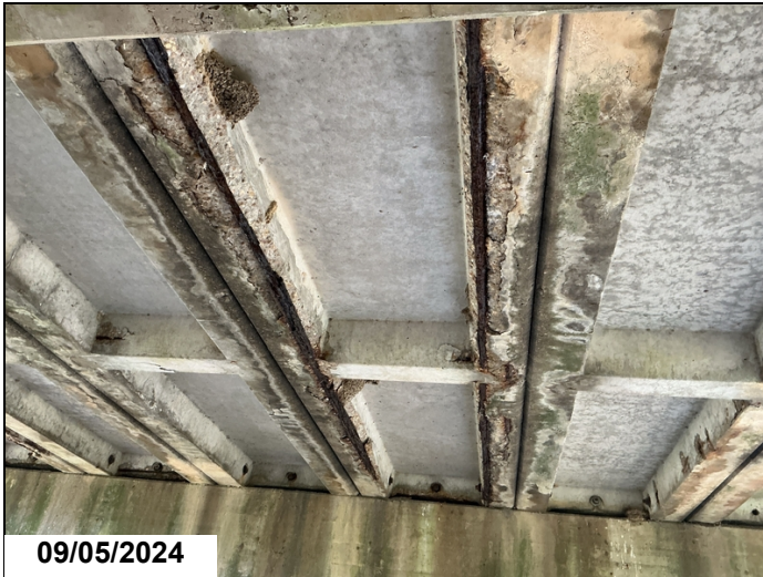
Exposed rebar left and right leg unit 5 span 2.
