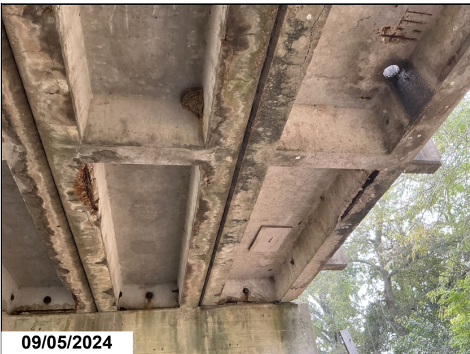
Exposed rebar left leg unit 6 and right leg unit 7 span 5.
