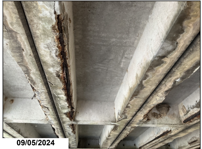
Exposed rebar to left leg unit 3 span 6.
