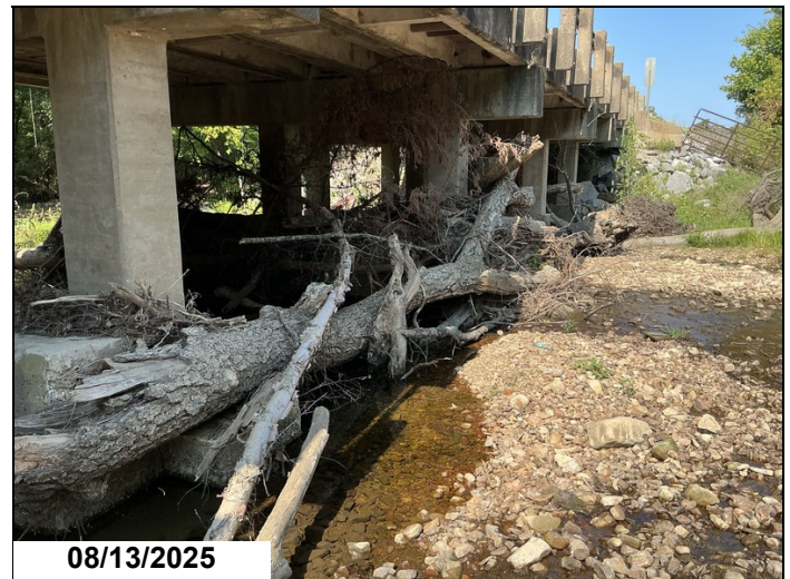
Drift @ Spans 1 - 5. Beginning to cause local scour.
