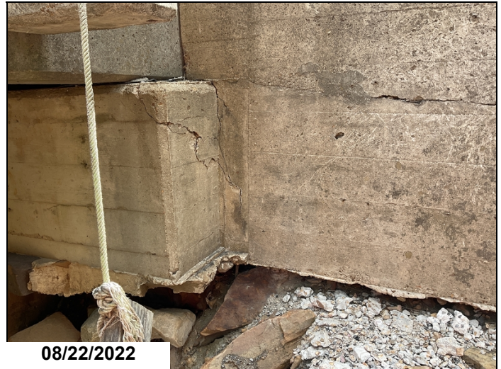
Erosion to Left & Right wings @ Abutment 2 with Left wing starting to crack.
