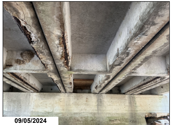
Exposed rebar to left and right leg unit 5 span 6.
