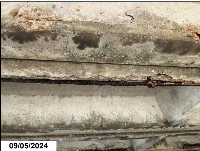
Exposed rebar right leg unit 6 span 6.
