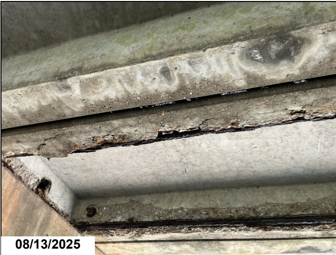
Units that have spalls with rebar exposed that have lost adhesion to concrete: Span 1 Unit 6.
