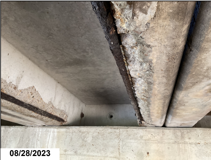
Spalls with rebar exposed with heavy s/l to Girder 4 @ Span 6. 4' of rebar is not adhered to concrete.
