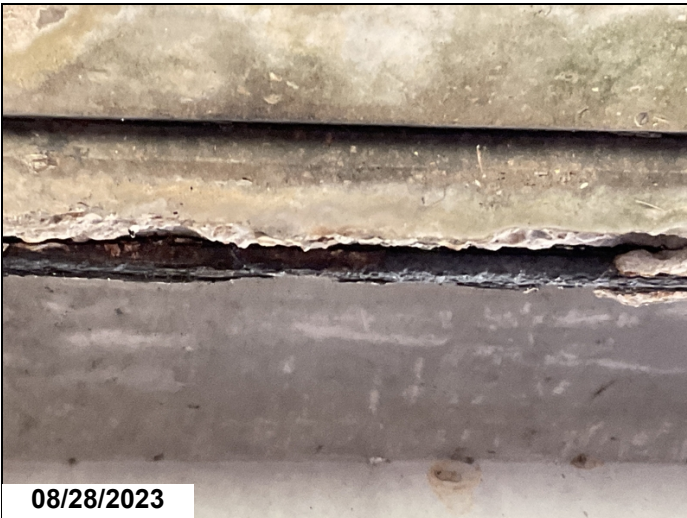
Spalls with rebar exposed with heavy s/l to Girder @ Unit 5 @ Span 3. 3' of rebar is not adhered to concrete.
