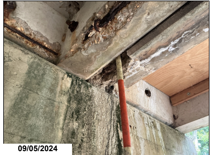
Deep spall right leg unit 1 span 6.
