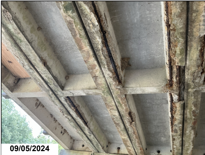
Exposed rebar left leg unit 2 and left and right leg unit 3 span 5.
