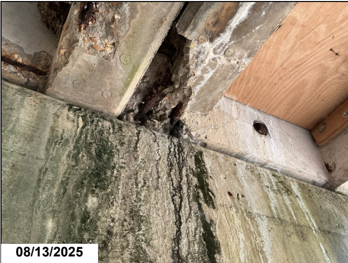
Spall with exposed rebar to right leg of unit 1 beginning of span 6.
