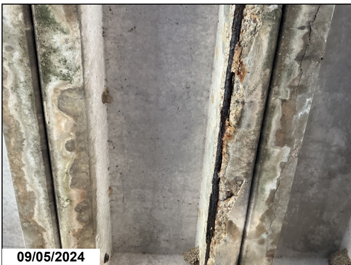
Exposed rebar right leg unit 3 span 3.
