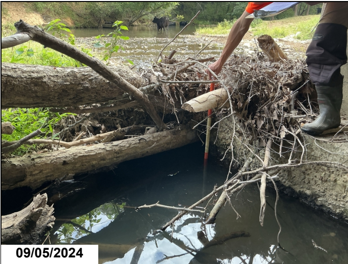
Scour 2' down 1' under bent 4.
