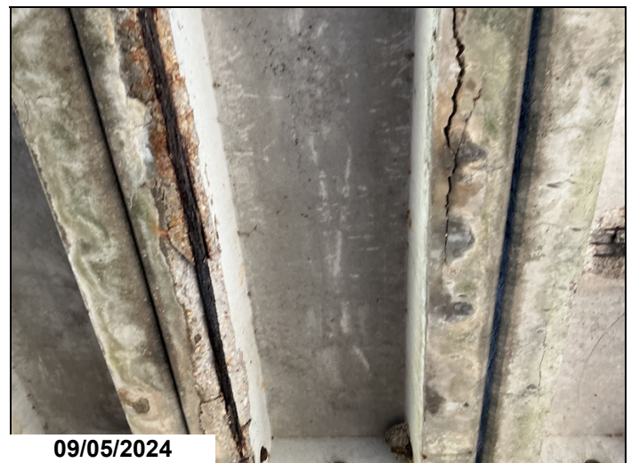
Exposed rebar left leg unit 5 span 3.
