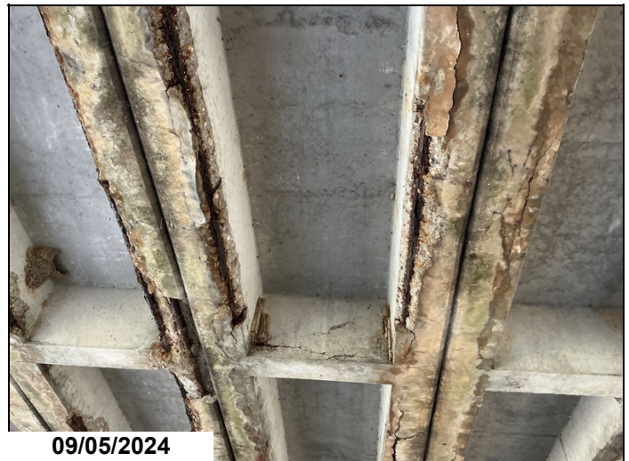
Exposed rebar to left and right leg unit 4 span 5.
