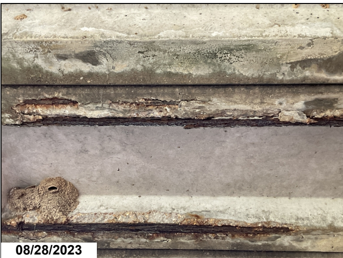
Spalls with rebar exposed with heavy s/l to Girder @ Unit 5 @ Span 2. 10' of rebar is not adhered to concrete.
