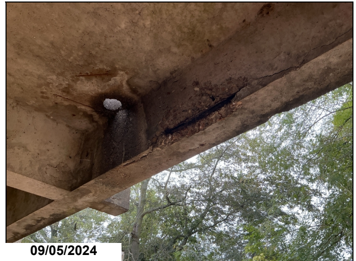
Exposed rebar right leg unit 7 span 6.
