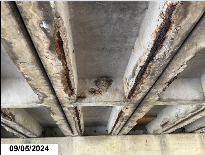
Exposed rebar to left and right leg unit 4 span 6.
