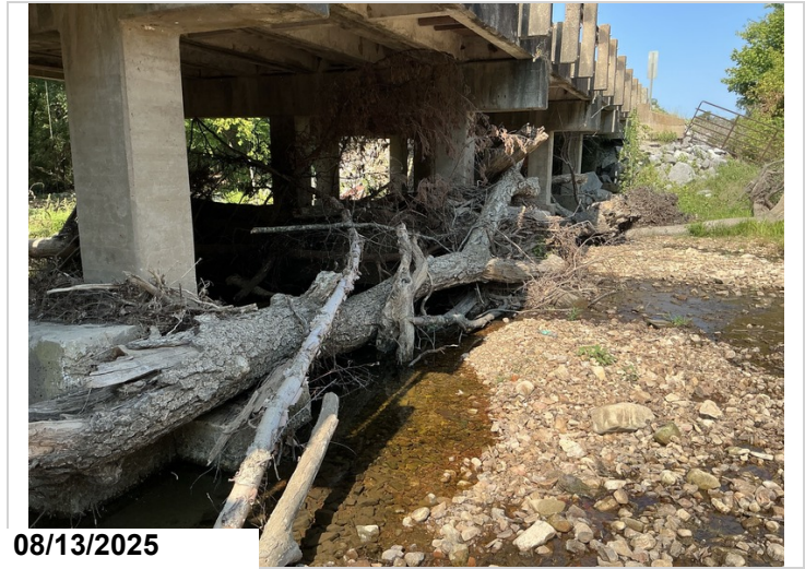
Drift @ Spans 1 - 5. Beginning to cause local scour.
