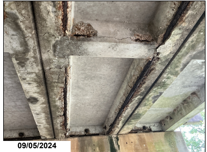
Exposed rebar left and right leg unit 6 span 1.
