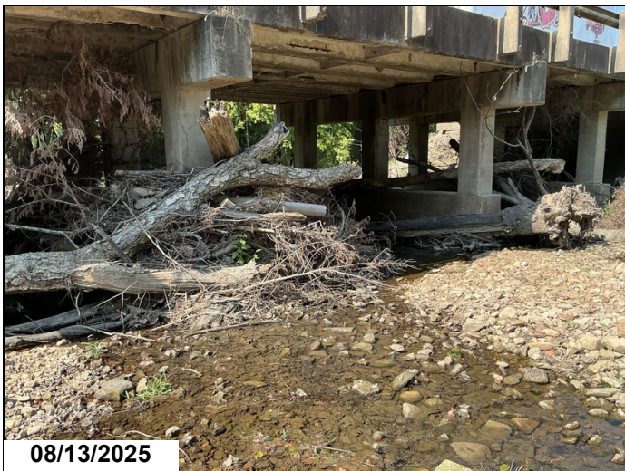
Drift @ Spans 1 - 5. Beginning to cause local scour.
