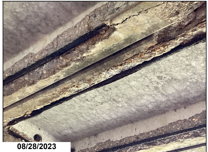
Spalls with rebar exposed with heavy s/l to Girder @ Unit 2 @ Span 2. 7' of rebar is not adhered to concrete.
