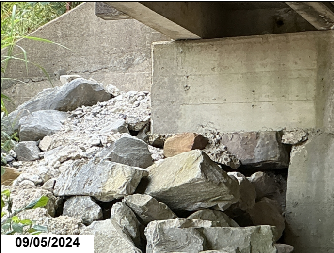
Erosion to wing and left side of abutment 2.
